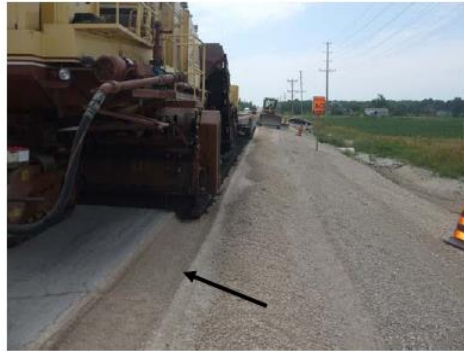
Pavement widening trench for CIR paving to extend under PPS.
