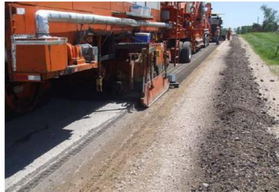
Straight, clean, vertical trench created for widening.
