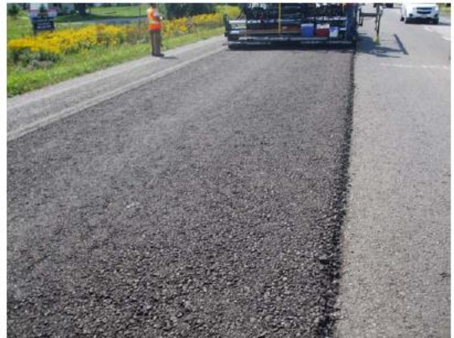
Coarse, segregated areas noted in mat behind CIREAM paver.
