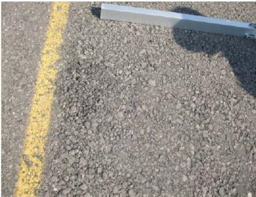
Close-up of loose, coarse mat at centreline. Material was kicked up easily with boot.
