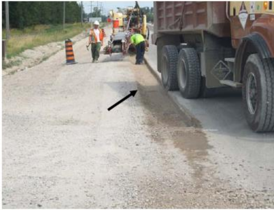
Excavation for pavement widening performed with milling machine. Trench with mostly straight, vertical faces.
