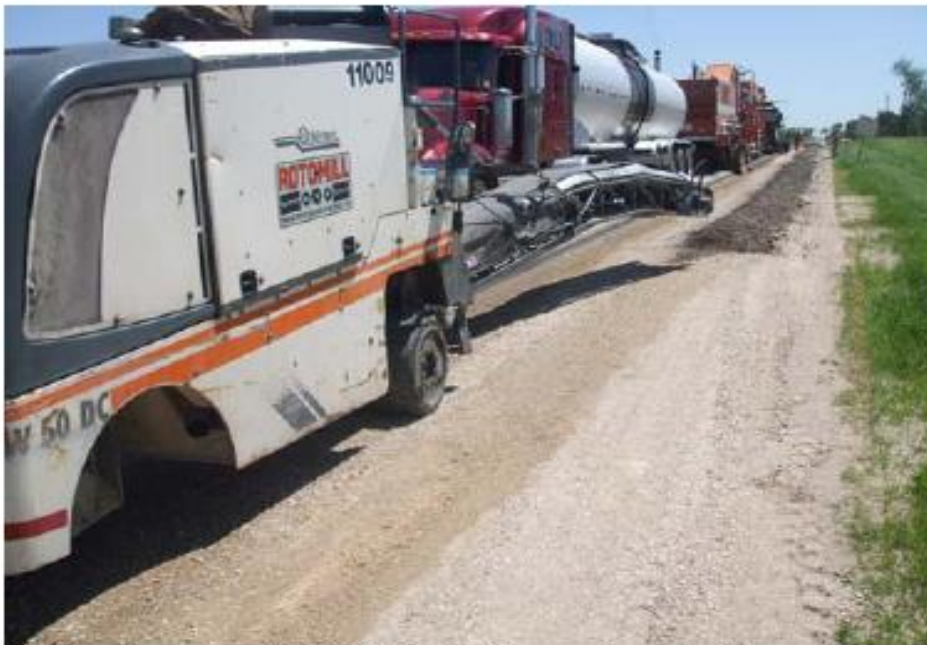
Widening for CIREAM PPS performed by milling machine.
